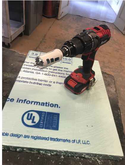
Image 39. Drill and 7/8” attachment for drilling holes in insulation board
