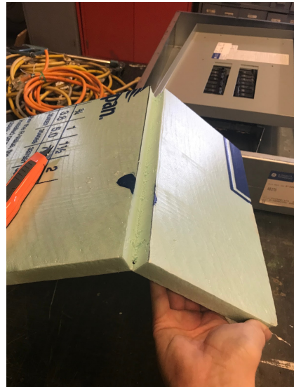
Image 37. Using a box cutter to cut insulation Image 38. Breaking apart insulation board
